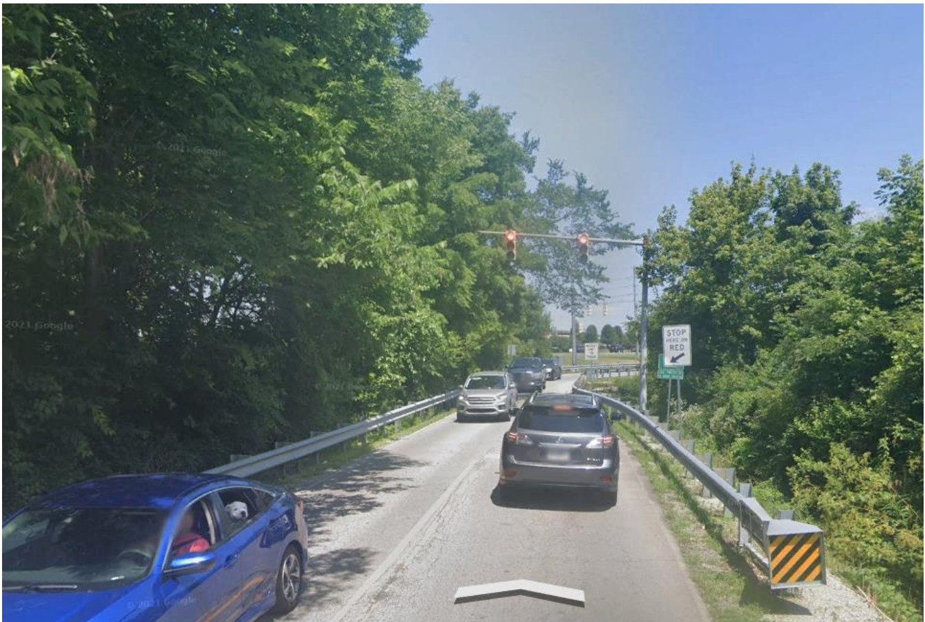
Figure 2 Example of Signal Controlled Single Lane Bridge
